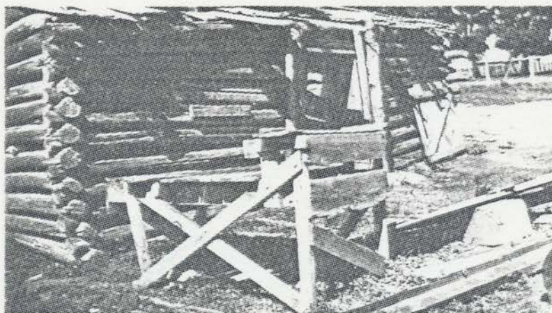
Remains of one of the little log cabins erected for the John Shawcroft family in Richfield in 1883.
